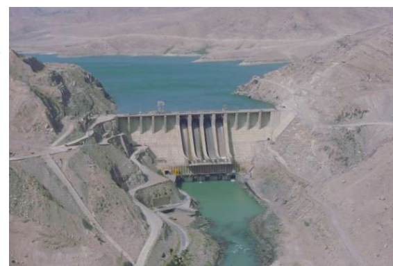
Why is the area around this dam so barren?
